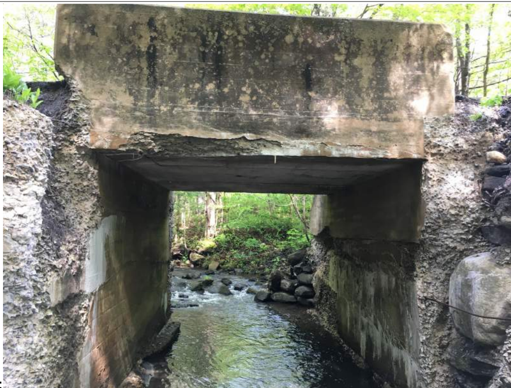
ii. Culvert Inlet:
