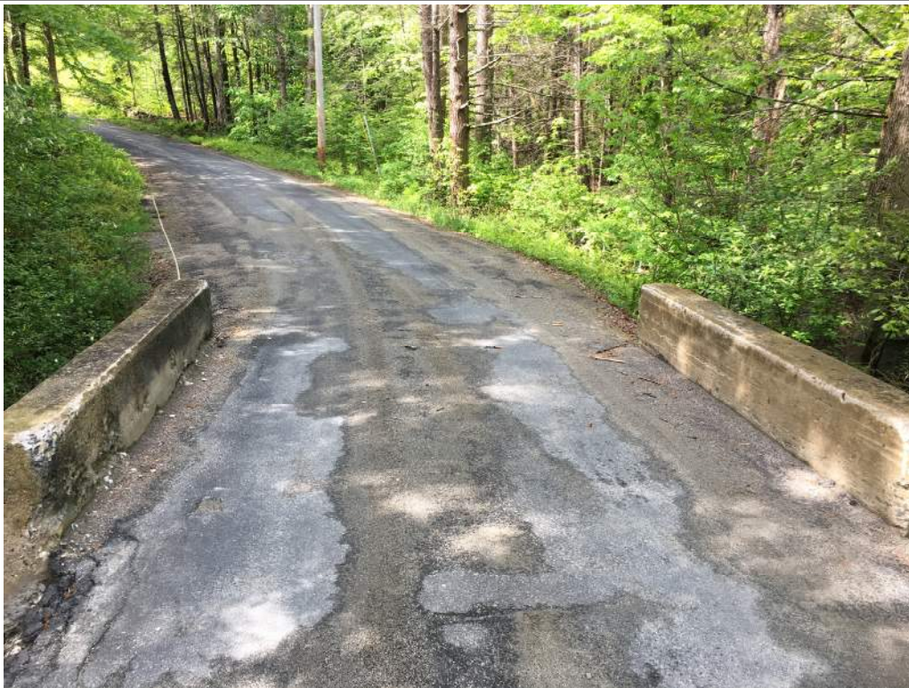
i. Road Over Culvert:
