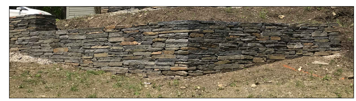
ASHFIELD STONE WALL CHARACTER
