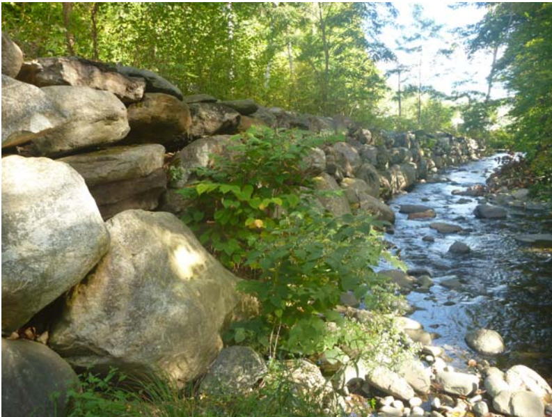
Figure 15 - Bank armoring along Clesson Brook includes a) boulder riprap, b) gabion baskets, c) stacked boulder walls, and d) concrete retaining walls.
