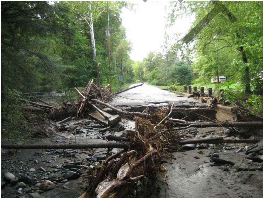
Figure 11. Photos of the aftermath of Tropical Storm Irene show a) extensive damage to paved surface of Clesson Brook Rd, and b) channel cutting through bridge crossing on Clesson Brook Rd (photos courtesy of Andrea Donlon).
