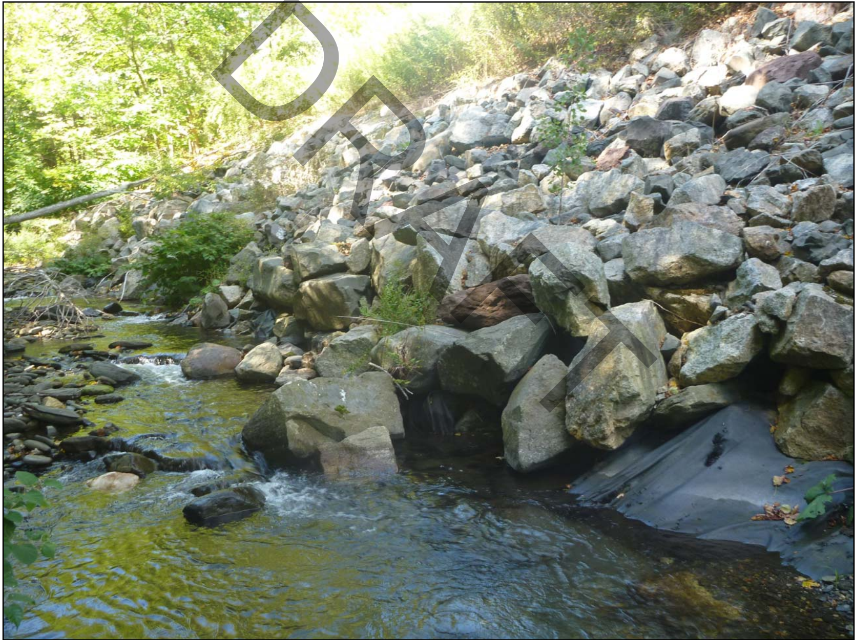
Figure 16. Upstream view of headcut undermining boulder riprap along Clesson Brook Rd.
