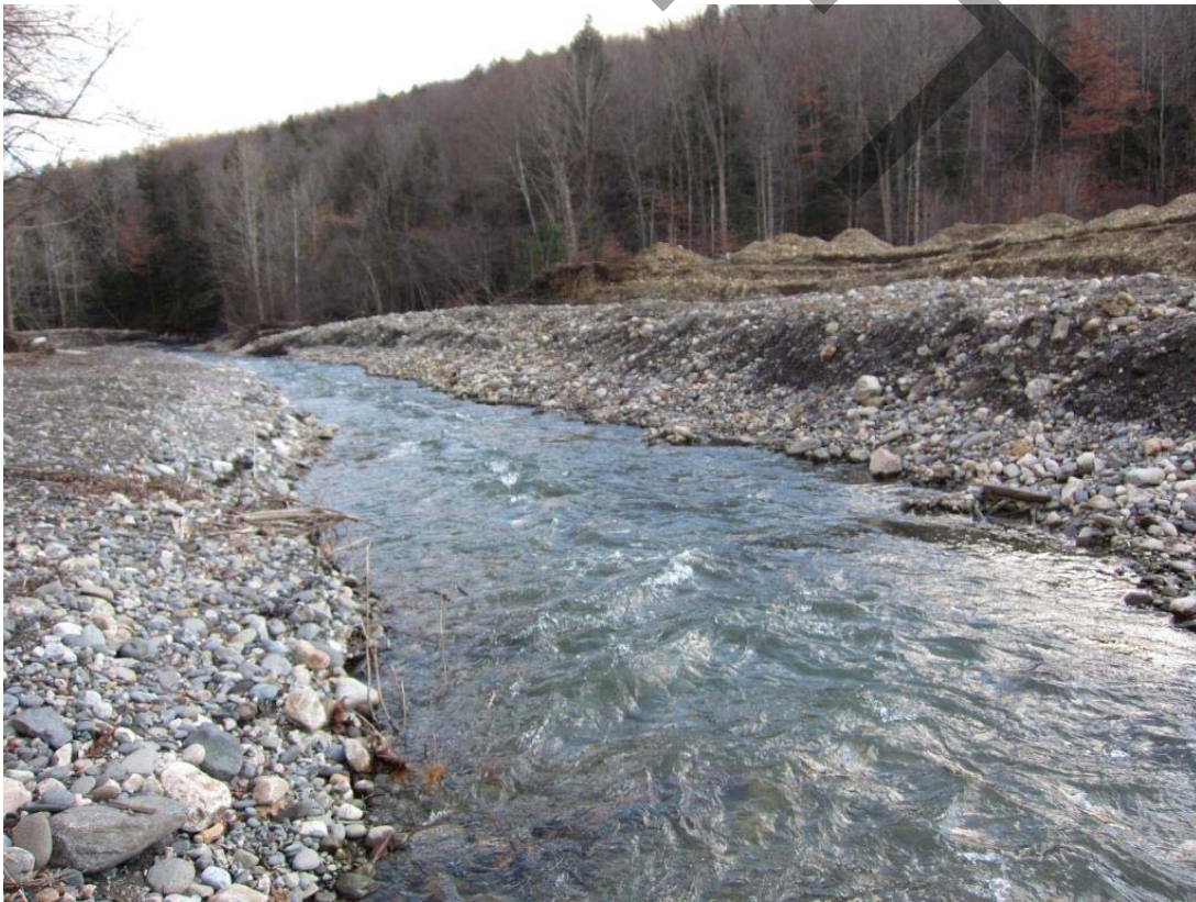
Figure 12. Emergency work completed in the months following Tropical Storm Irene included extensive windrowing, as gravel and cobbles were excavated from the channel and piled as berms along Clesson Brook (photos courtesy of Andrea Donlon).
