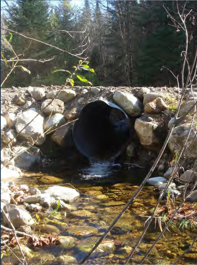
Before – October 2012 (looking upstream) 4' diameter CMP; 0.6' drop
