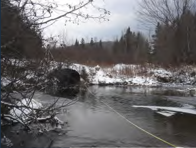
Before – Nov. 2013 (looking upstream) 6.25' diameter steel culvert; 40° skew
