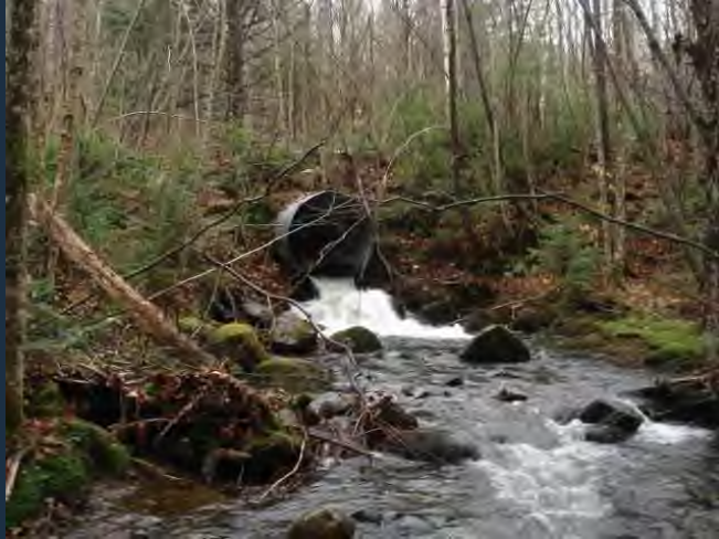
Before (looking upstream) 5' diameter CMP; 2.8' drop
