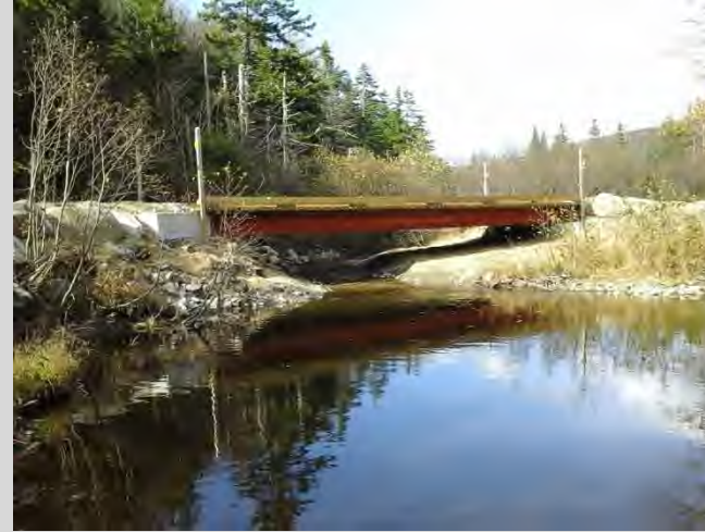
After – Oct. 2014 (looking upstream) 46' clear span; steel beam bridge
