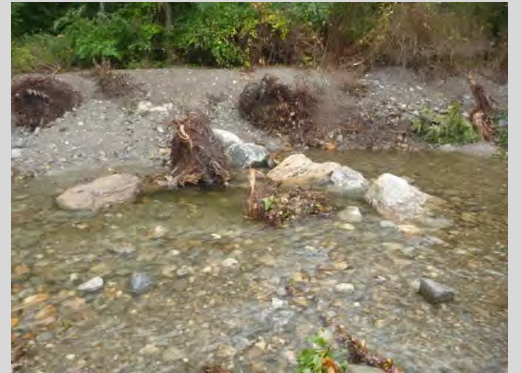
Example of a completed restoration project: boulder deflectors positioned in stream to help slow the flow
