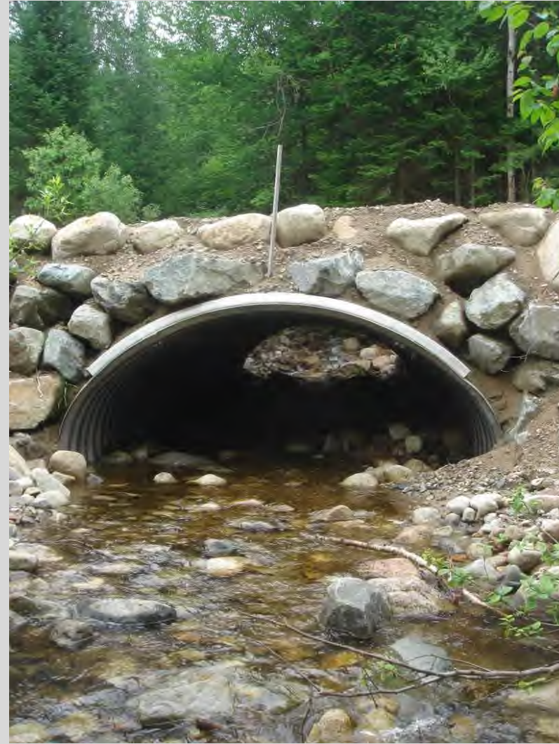
After – July 2013 (looking upstream) 10.75' embedded aluminum arch
